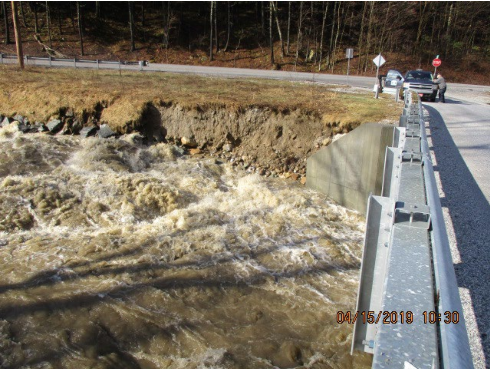
Town Bridge #25 on Medway Road over Mendon Brook – April 2019 (DR4445)
