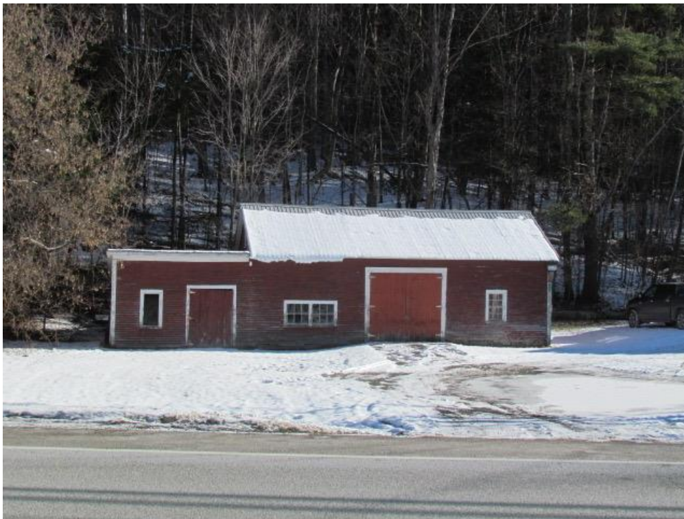
Photograph 8: 1990 US Route 4 Barn
